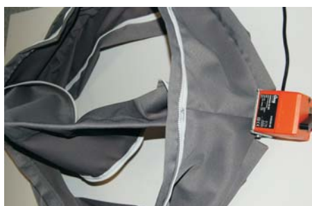
Flap and servomotor detail
