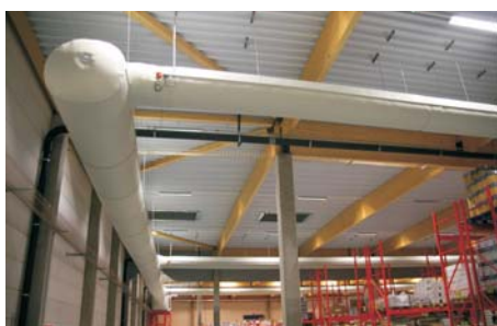
Installation of membrane diffuser
