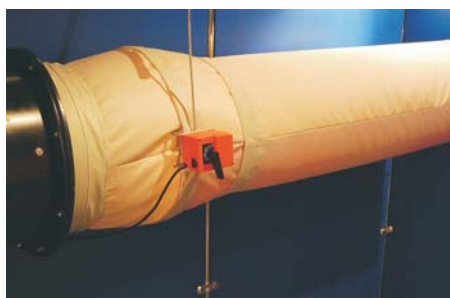
Detail of servomotor installation
